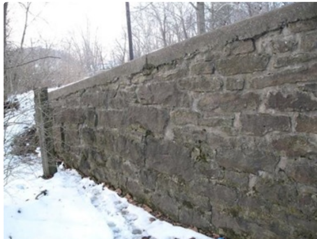
Freestanding and splayed wing wall
