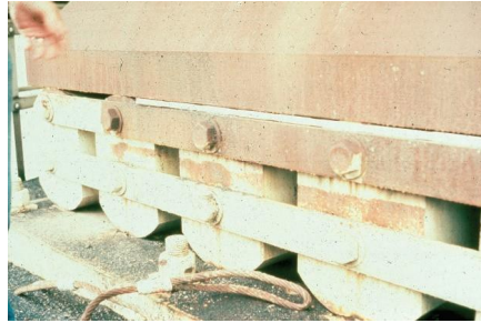
Segmental rocker nest bearing
