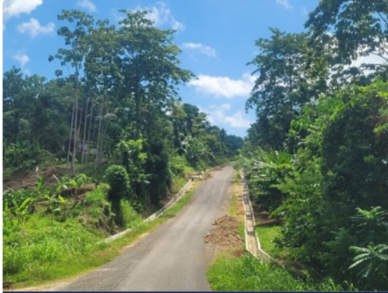
Type 5 Open drain on both sides of the road on New Britain Highway, East New Britain
