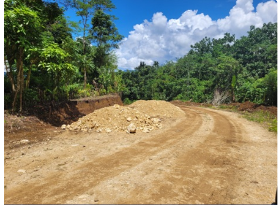
Excavation and widening along the New Britain Highway, East New Britain
